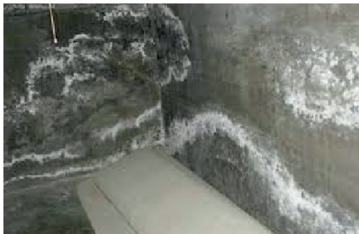
Salt Efflorescence
