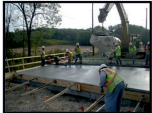
Figure 5: Internally Cured Concrete Bridge Deck being Cast Near Bloomington, IN (Di Bella, Schlitter, & Weiss, 2010)
